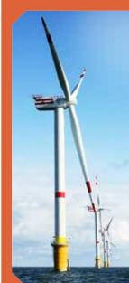
Some wind turbines are in the middle of the ocean! These wind turbines collect energy out at sea and transfer the energy to places on land through huge underwater cables. This is called offshore energy.
