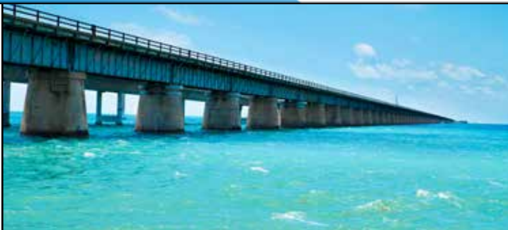
The Seven Mile Bridge in the Florida Keys is an example of a beam bridge.
