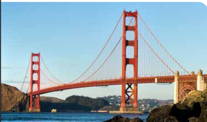
The Golden Gate Bridge in San Francisco is an example of a suspension bridge.
